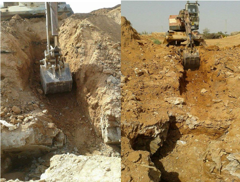
Figure 21. Digging trenches with a backhoe at Meshrefet Anz (photo taken by a volunteer team member on 12 September 2015).
